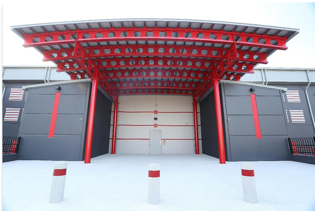
Data Center- Head Office
